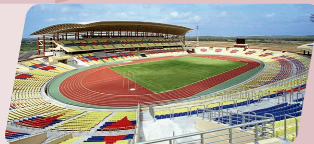
Hang Jebat Stadium, Melaka/Malaysia (MX system family)
